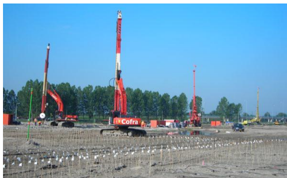
Figure 10. Installation of the vertical drains
