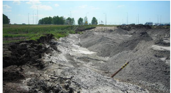
Figure 7. Squeezing of the peat under the placement of the sand
