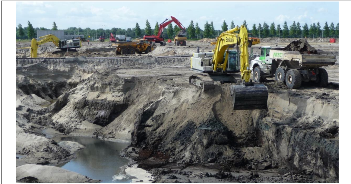
Photo 2: Photograph of the excavation of the compressible layers underneath the sand layer
