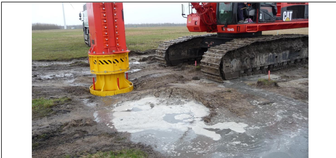
Photo 1: Compaction of a trial location. Note the subsidence on the surface and the water in the previously compacted location
